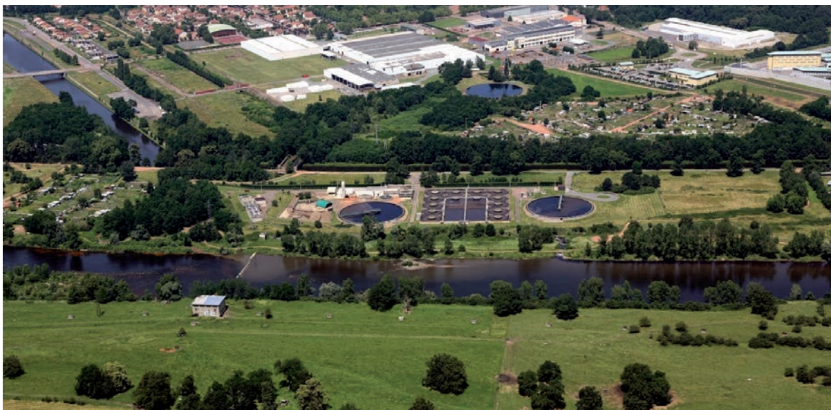
Station d'épuration – Roanne
